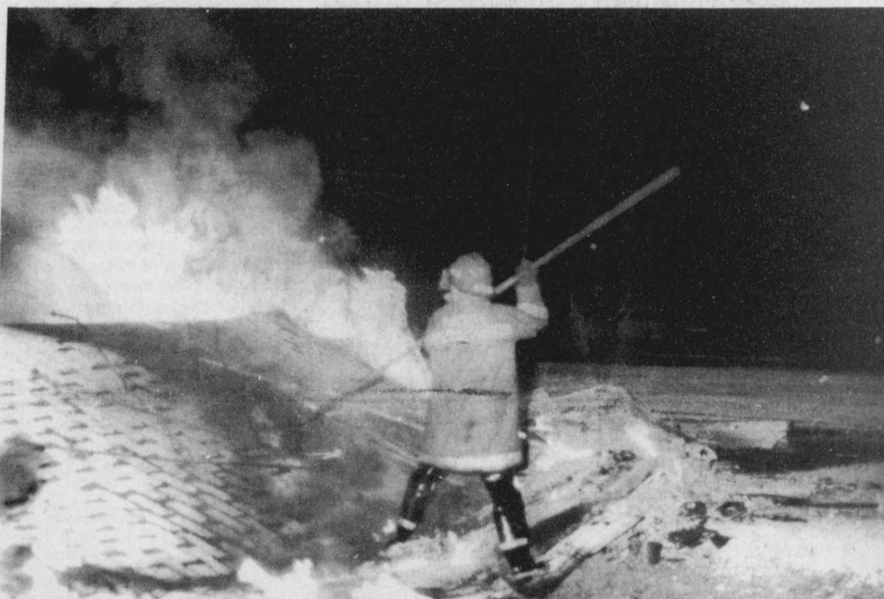
UPIN SMOKE -The older scale house at Blackland Prairie Gin was torn down and the Deport Volunteer Fire Department
