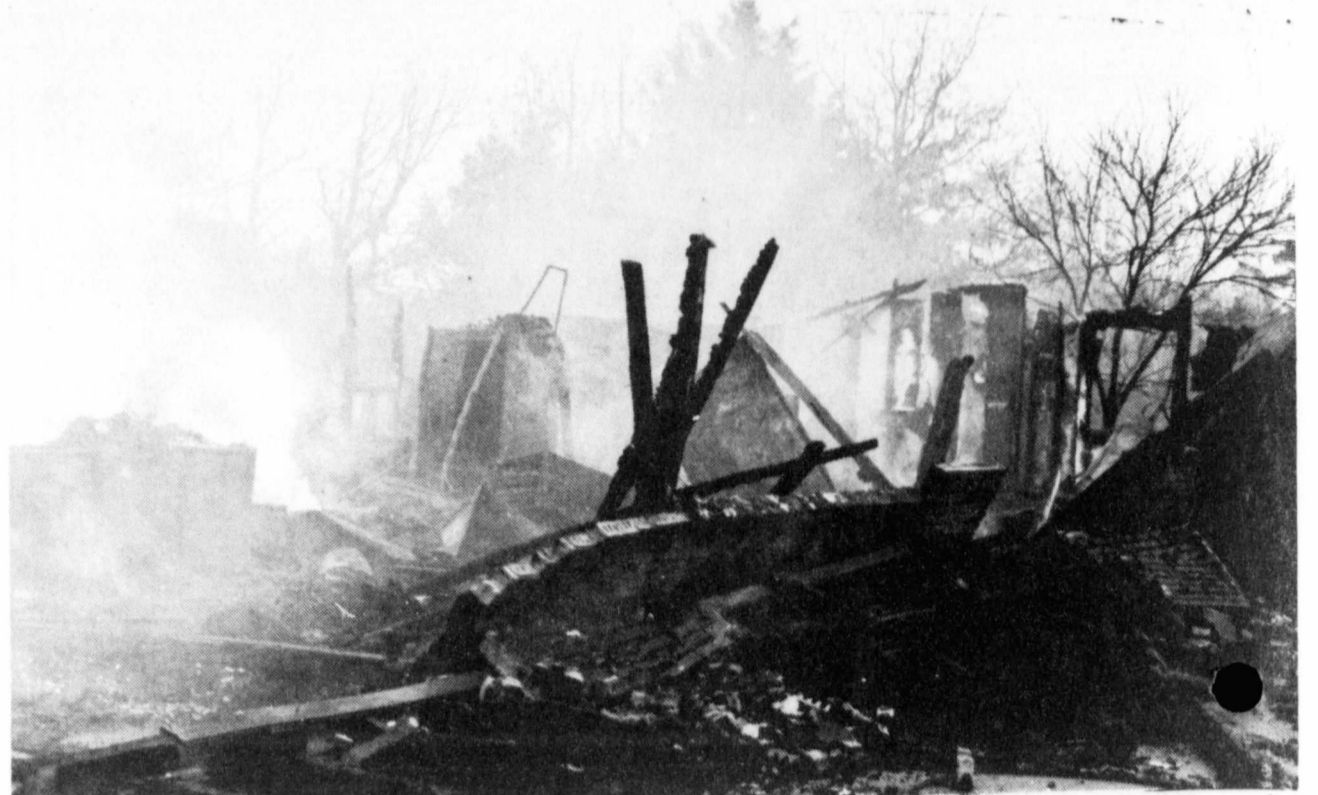
DESTROYED -The home of Jerry and Cherrie Gillie of Sylvan was totally destroyed by fire last
