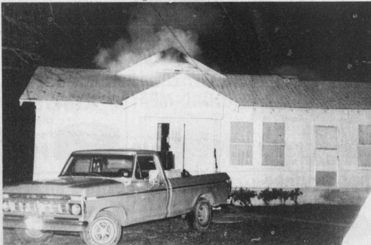
DAMAGED-The home of the Ricky McMikel's was damaged in the attic by fire that started from
