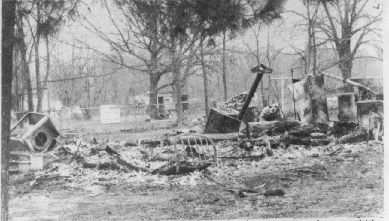
COMPLETELY Destroyed—This home belonging to Freddy Anderson of S. Bois D'arc in Blossom was completely destroyed by fire. The Blossom
