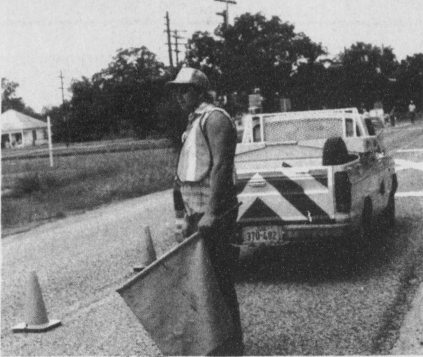
STRIPING the road—Old Highway 82 has been recently resurfaced in Blossom and Jessie Lullie has been busy painting railroad crossing stripes back to their original form. (Staff Photo by Charlene Barker)
