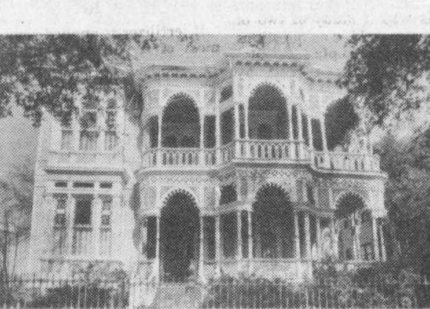
QUEEN CITY OF THE SOUTH... Galveston, Texas, is nationally known for its Victorian architecture. Shown is the famous Sonnetheil House built in 1886.
