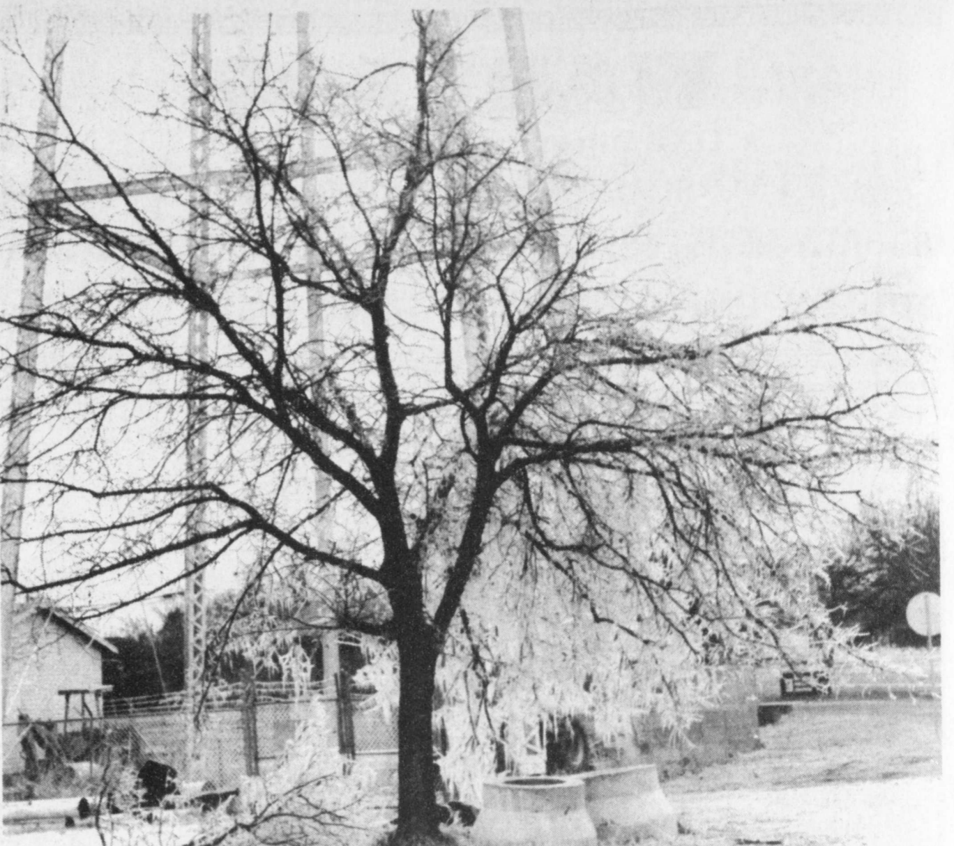
FROZEN—The cut-off valve adjacent to the Blossom water tower was frozen, causing problems in the area. (Staff Photo)
