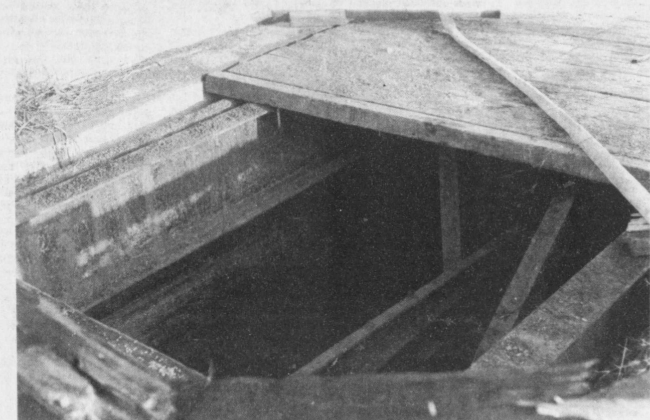
BREAK THROUGH-the scales at the Blackland Prairie Gin in Deport are in for some major repairs after a truck driven by C.R. Williams and loaded with milo crashed through them last week. The milo had to be unloaded by hand wrecker removed the truck. (Staff Photo)
