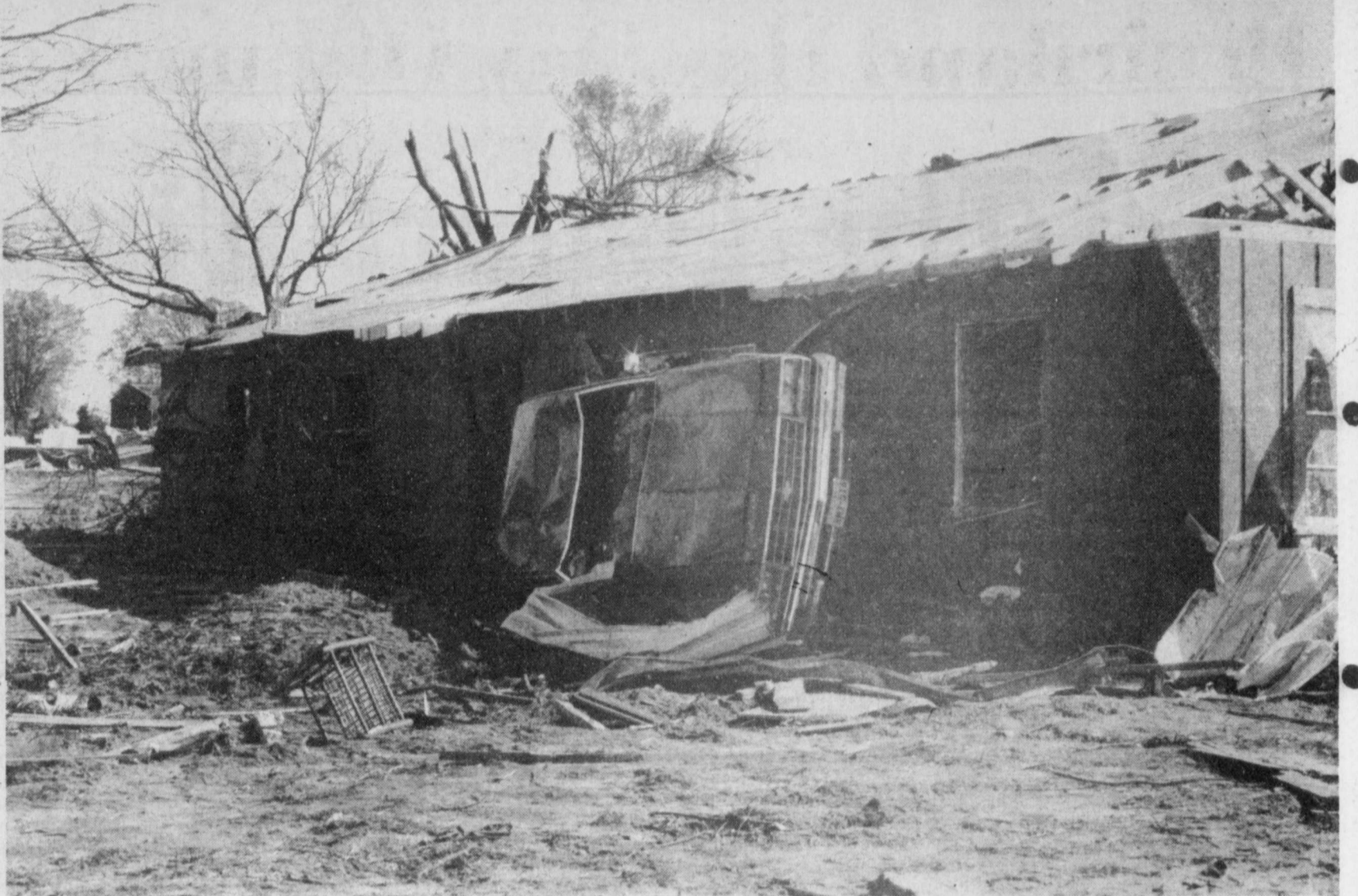
TORNADO damage—This house and car, belonging to the Crites of Blossom, was nearly destroyed by the tornado that swept through the area Friday. The Crites had only been in their home three days when the storm struck. (Staff Photo)
