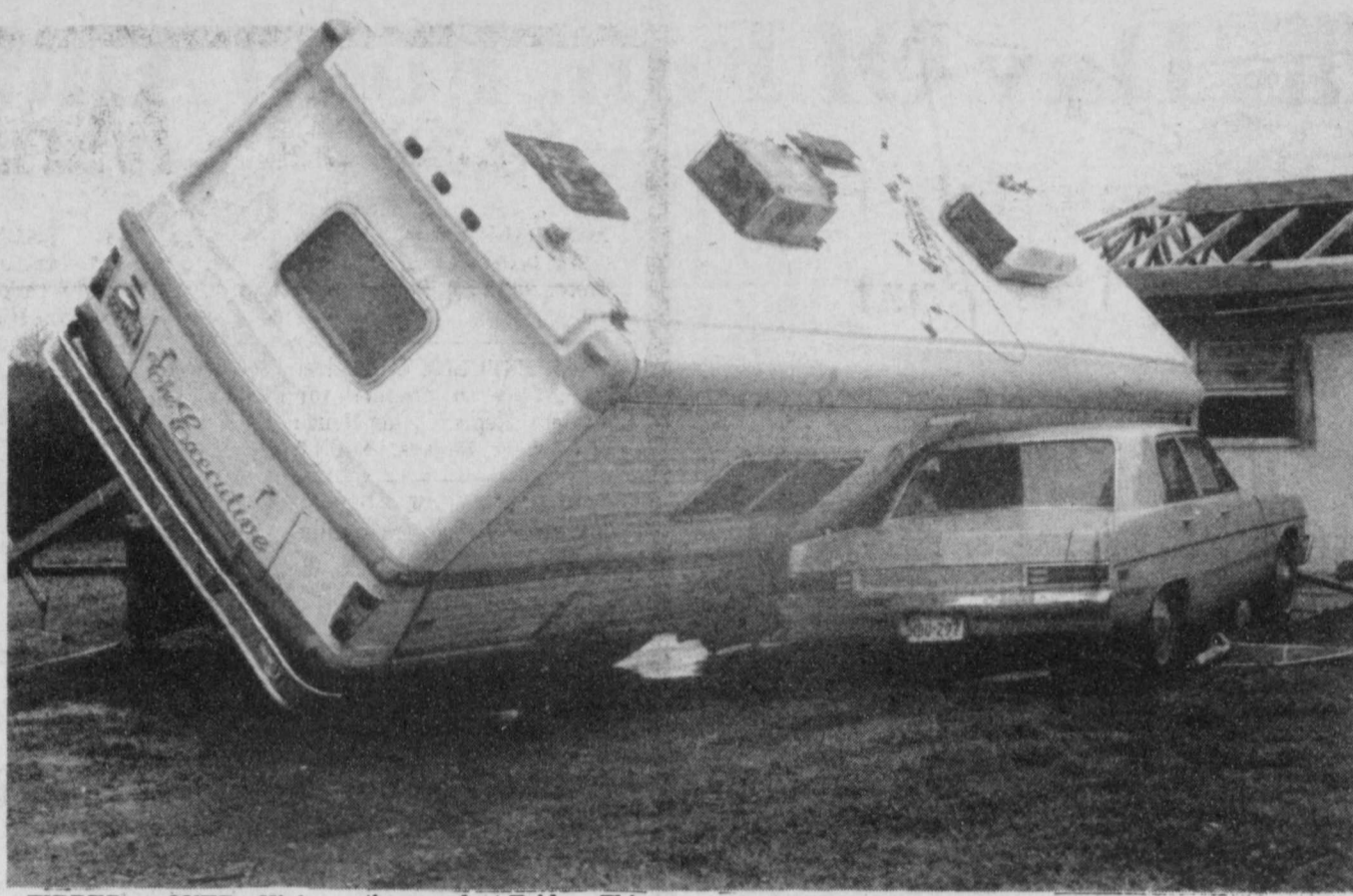
TIPPED OVER —High winds and incredible force accompanied the tornado that devastated the area last Friday. This camper, belonging to Ann Dudley, was tipped over onto the family car, while the house suffered severe damage. Neighbors have teased folks about their "odd ways to park". (Staff Photo)
