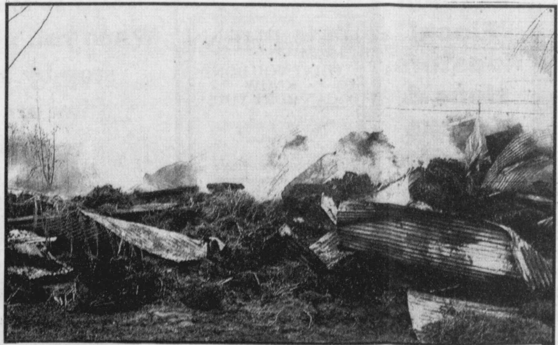
FIRE-swept through the old buildings behind the main street in Talco Wednesday night destroying them almost completely. The buildings belonged to Mr. and Mrs. Gene Smith of Talco and were formerly the out buildings of Jack Winn's store and later Smith's Hardware and Propane. The blaze is suspected arson. (Staff Photo Nancy Brown)
