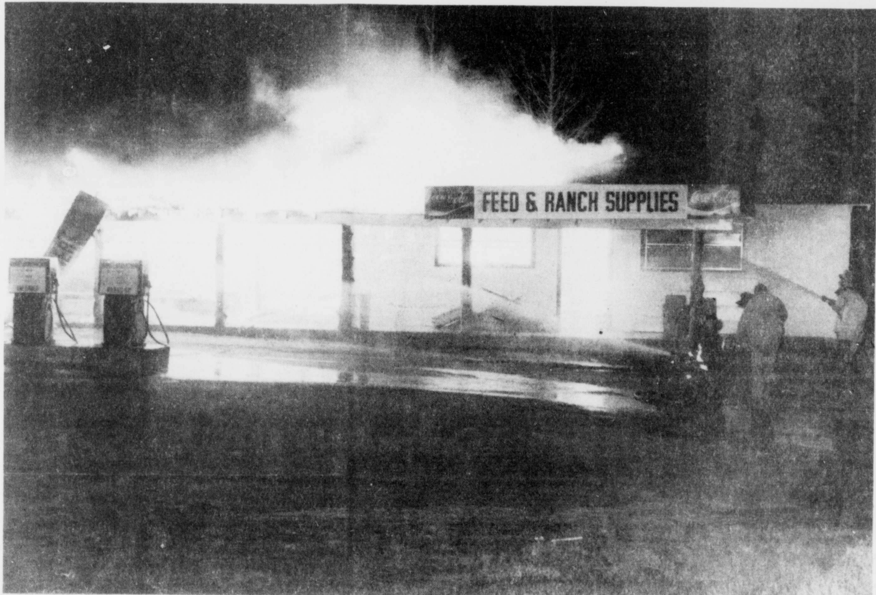
DESTROYED—Jim's Country Corner grocery was totally destroyed by
