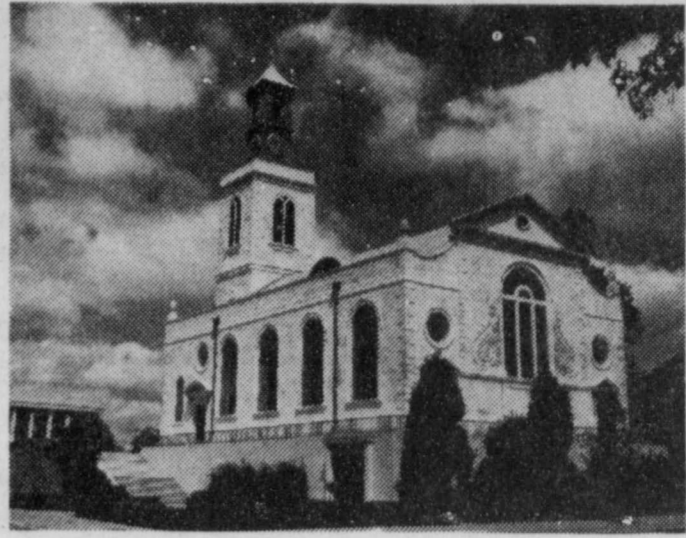
REASSEMBLED . . . The 12th century church of St. Mary Aldermanbury was brought from London in pieces and reassembled on the campus of Westminster College in Fulton, Mo.
