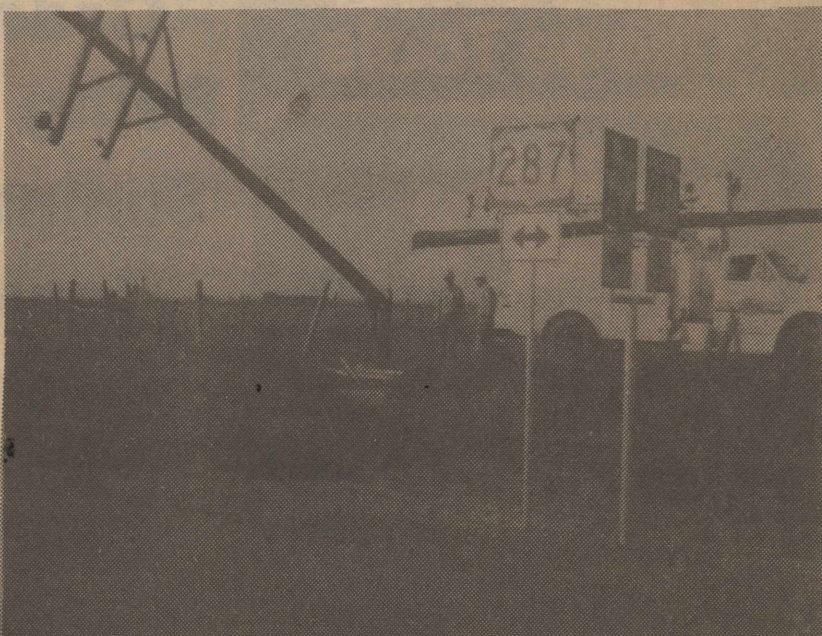
A wheel came off a truck last Wednesday afternoon, in Kerrick. A SWPS crew was out to replace the broken pole at the intersection of highway 287 and FM 807. At first it looked as if someone hadn't made the stop sign from 807 as the pole is located directly across the road. Fortunately, no animal or person was in the wheel's path!
