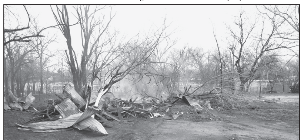
HOUSE DESTROYED-A vacant house in the 900 block of South First in Haskell was totally destroyed by fire late Tuesday night, Feb. 19. The fire caught in the trees and grass on the south side of the creek. Haskell fire department members contained the fire and city employees helped with the debris.
