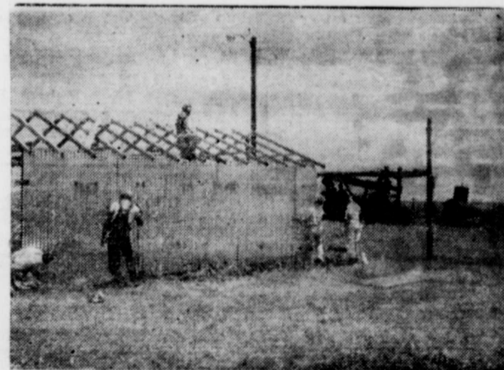
EVERY NAIL HELPS TO COMPLETE THE BLACKSMITH SHOP . . . FOR THE FUTURE
