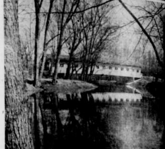
COVERED BRIDGE that combines the authentic rusticity of colonial America with the latest in modern design and materials has been erected over the Sanga-mon River in Illinois. Steel girders are its main supporting members, lowering costs and simplyfying
