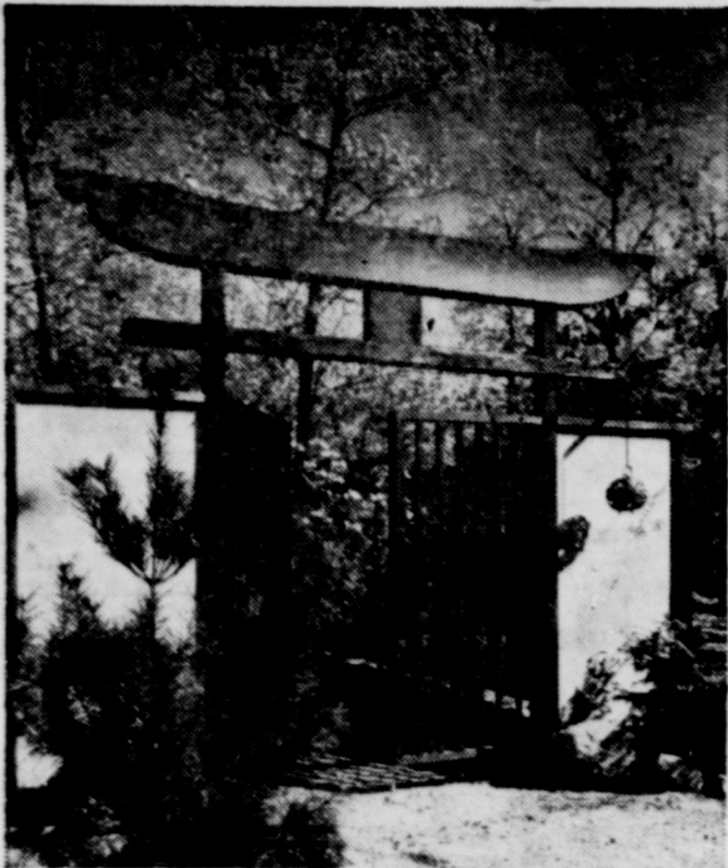
Oriental influence on American architecture is becoming more pronounced. The design often is from the East while the materials are native to the United States. In the photograph above, the garden gate is an adaptation of a Japanese Shinto shrine entrance. The fence is made of natural-color, whitish mineral fiber sheets, an inexpensive, easily maintained material that contrasts handsomely with the redwood framing to which it is nailed. Pre-finished sheets in other colors could be combined with painted frames to give many different effects.
