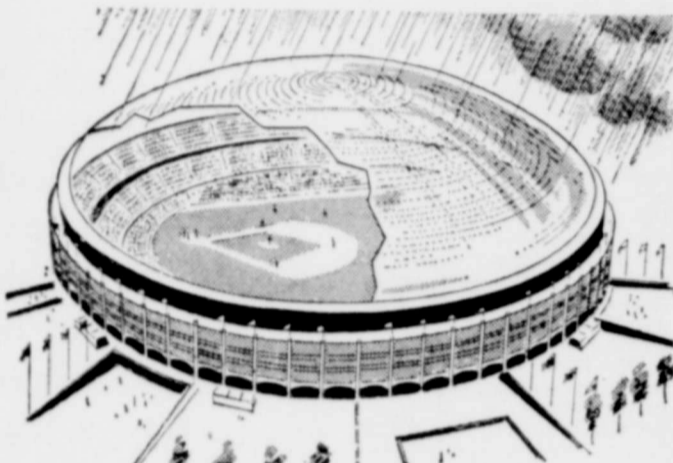
It'll be a rainy day in Texas and a great day for a baseball game at Houston's Harris County Domes Stadium, the world's first indoor-outdoor weatherproof sports arena. Only the sun will be able to penetrate the skylight roof of Du Pont's "Lucite". Inside the stadium 2 1/2-million cubic feet of air will be cooled and circulated each minute.
