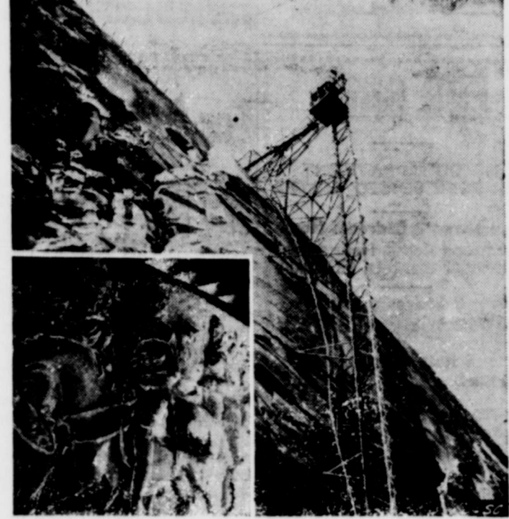
Using sturdy modern steels and plenty of patience, stone cutters are carving three Confederate heroes—Robert E. Lee, Jefferson Davis and Stonewall Jackson—into the side of an 870-foot mountain near Atlanta, Ga. Working on a platform atop 270-foot hoist made of strong steel pipe and angle framing, the men are sculpting the 145 x 195-foot bas-relief shown in plaster model (inset).
