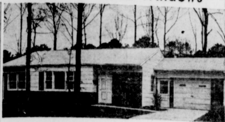
John Aragona, builder of this home in Norfolk, Va., found that wood, with its natural richness, has a strong appeal to home buyers. He switched to wood windows and stepped up sales in the $96 million Princess Anne Plaza development almost overnight.
