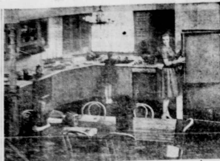
The kitchen is the first place to look for quality in a new house. This kitchen, with its ample cabinet space and work-saving electric appliances, has a feeling of livability and warmth. Its extra living space easily accommodates a good size table for eating or homework.
