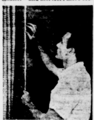
Measuring the rooms of a house is the first step in determining its heating requirements.
