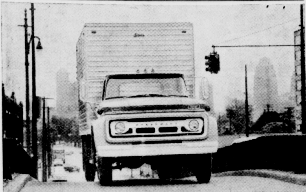
Diesel power for the first time, addition of two higher powered V8's, and lower hood lines for better road visibility highlight Chevrolet's 1962 trucks, tinted glass and sliding rear cab window truck line. New to most of the 19's models are for better ventilation. Proved independent front suspension is retained with improvements.
