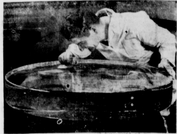
A TECHNICIAN examines the optical quality of a 36-inch telescope mirror that will ascend, by balloon, this year to 80,000 feet above the earth. The project known as STRATOSCOPE II will examine planets and galaxies. The disk, manufactured by Corning Glass Works, is made of fused silica, one of the purest materials known to man. The purpose of sending the telescope up in a balloon is to get it above the earth's atmosphere which obscures clear visibility of celestial objects. STRATOSCOPE II is supported jointly by the National Science Foundation and the Office of Naval Research.
