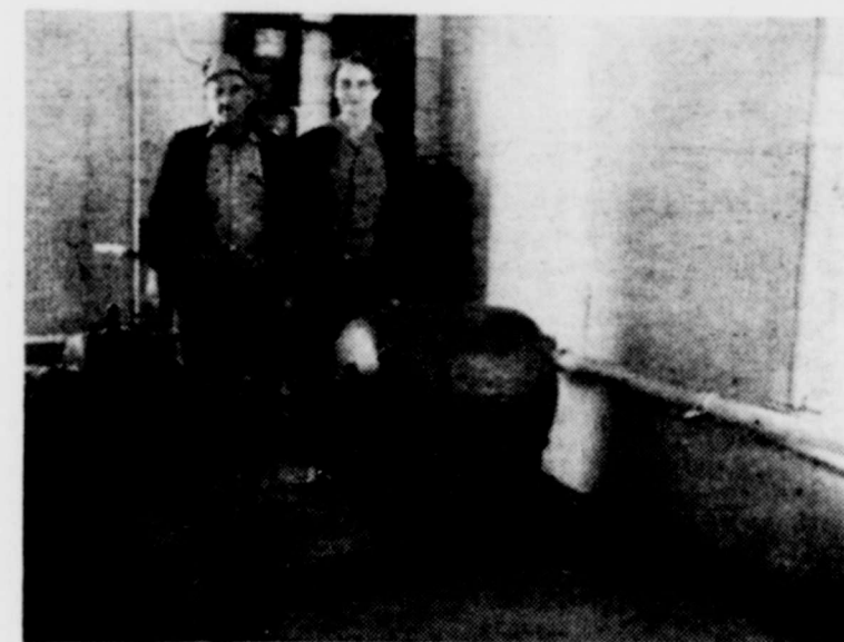
Mr. and Mrs. Jobie Dunn at one of the City's Water Pumps
