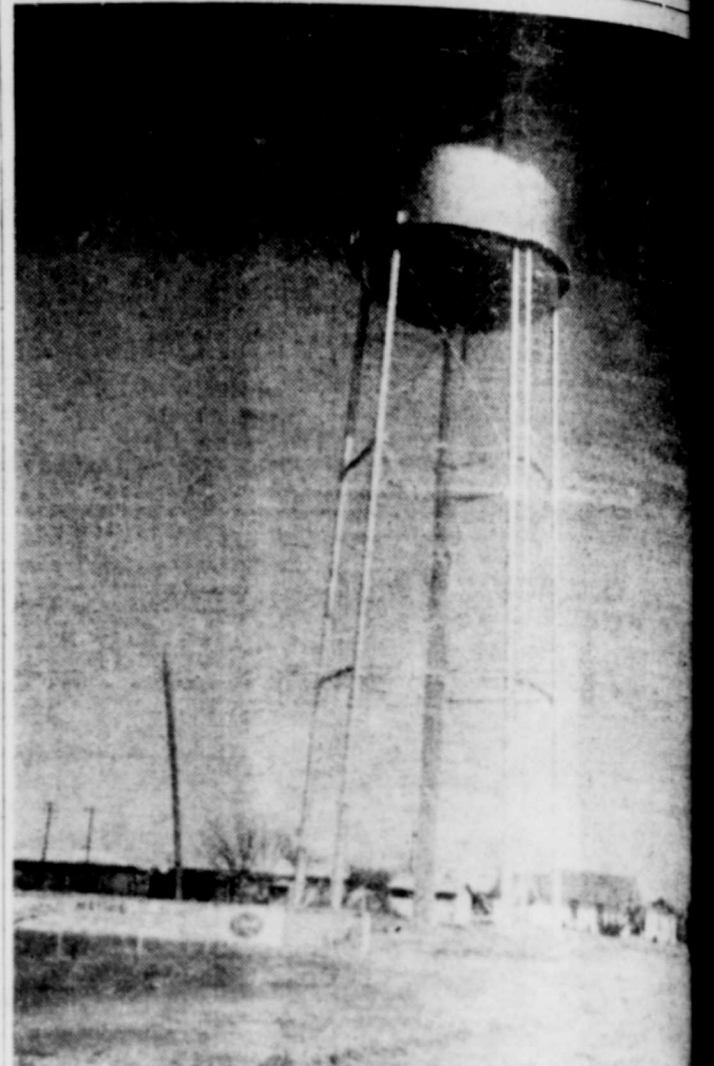
NEW WATER TOWER IN S-E PART OF CITY
