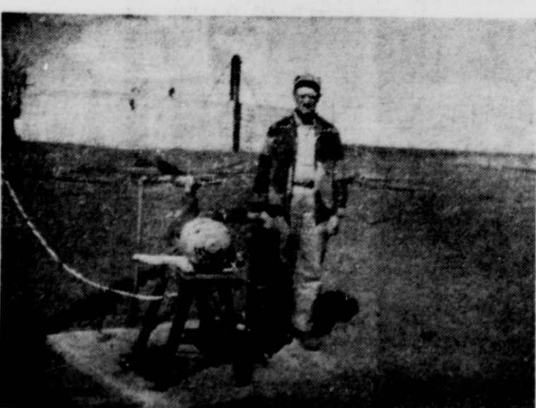
Fred Williams by one of the City's Water Wells
