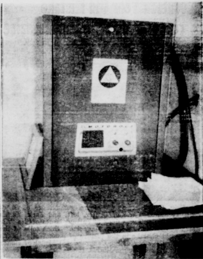
CIVIL DEFENSE BASE RADIO STATION
