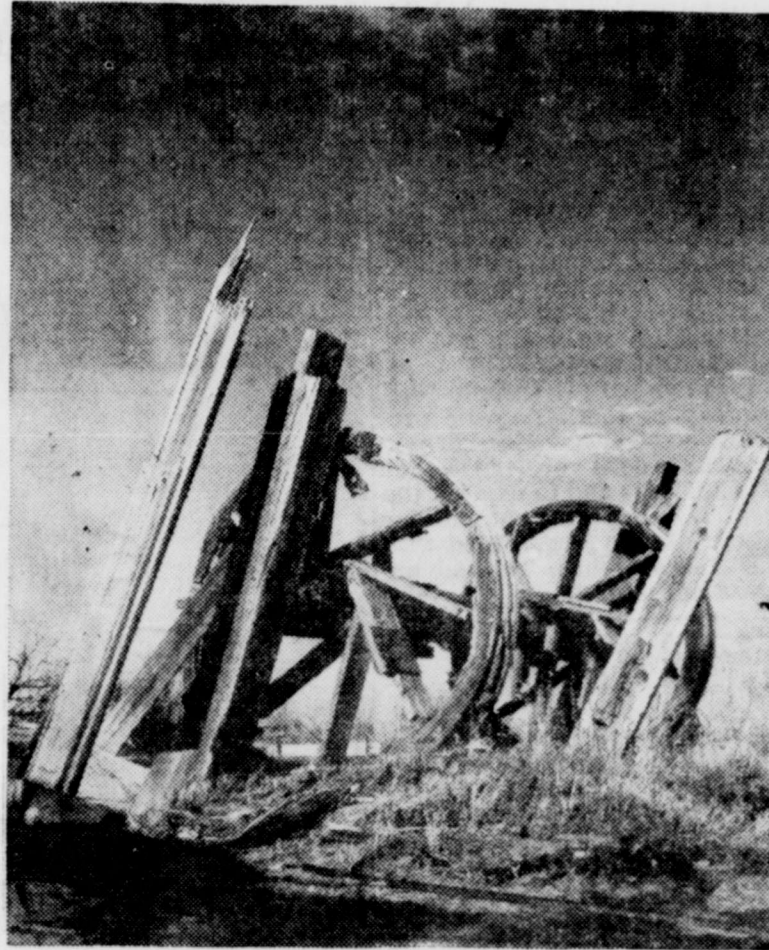
The broken remains of a wooden derrick, Burk-Divide No. 161, drilled in the early 20's, still point skyward from a point where the well once pumped crude oil from about 1500 feet in Red River bottom near Burkburnett.
