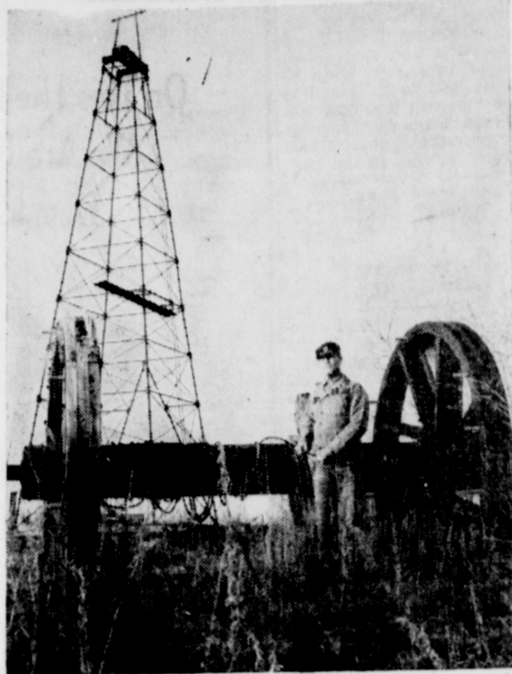
Newton T. Crane stands before some bull wheels which were used to help develop the Bridgetown Northwest extension of Burkburnett oil field. Reno No. 173, seen in background, is still producing. Crane, owner of the wheels and Reno No. 173, came to the area in the early 20's.
