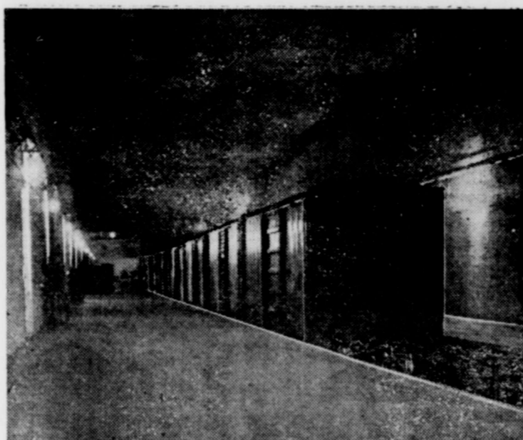
DEEP WITHIN a mountain in southwestern Missouri, freight cars await unloading of civil defense equipment to be stockpiled here for use in case of enemy attack. The siding, extending 600 feet into the mountain, can accommodate 16 railroad cars simultaneously. The Office of Defense and Civilian Mobilization facility, part of a limestone mine, contains a vast array of medical supplies and "hardware" to be used in recovery operations in the event of an attack on the United States. (Courtesy Southwestern Limestone Co.)
