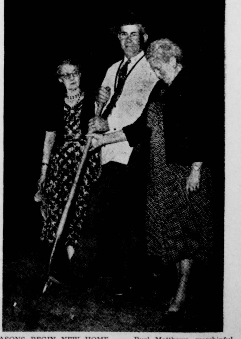
MASONS BEGIN NEW HOME — Burl Matthews, worshipful master of Burkburnett's Masonic Lodge, officially turned the first shovel of dirt for the construction of a new $35,000 Masonic building at Burkburnett Monday. Assisting are, left, Mrs. C. D. Scruggs, worthy matron of Eastern Star in Burkburnett, and right, Mrs. Hugh Jones, treasurer. The Lodge, No. 1027, was established Dec. 12, 1910. The new building will be constructed on Second Street and B. Avenue.
