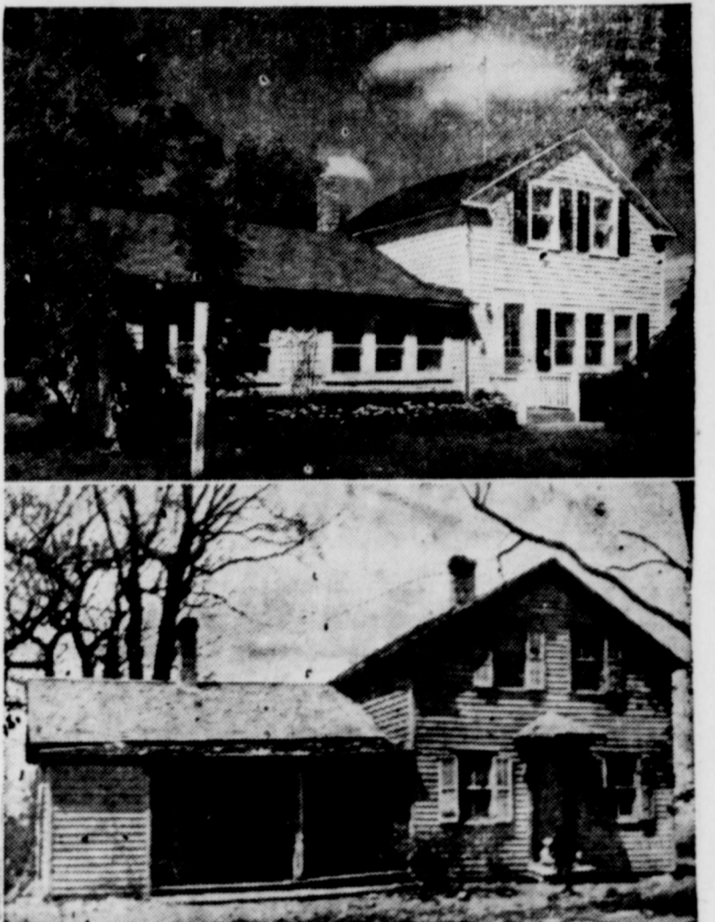
The handsome, new-looking home, top, is the remodeled version of the 100-year-old farmhouse, bottom. Window rearrangement, elimination of the porch, a new fire-resistant asphalt shingle roof, and new paint were principal exterior improvements.
