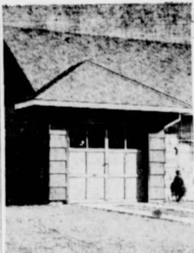
This garage is under the same roof as the house, but a hip roof-style projection over the garage adds variety to the design. Asphalt shingles are blended.
