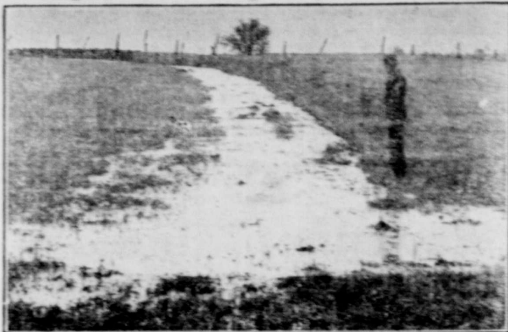
Terraces properly laid out and built will hold the water when it rains. Top soil will not wash away. Several miles of terraces have been built in the North Burk Conservation District in the past two years.
