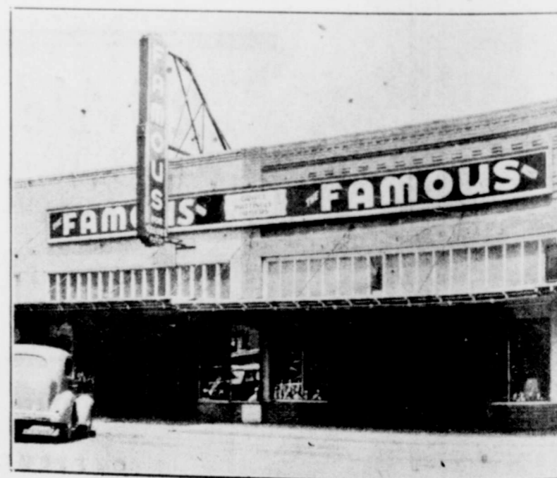
Present Location 50 Ft. Front
