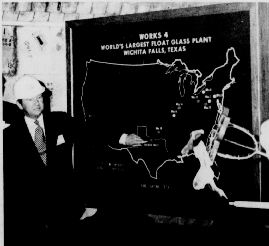
HEATS BRANDING IRON --U.S. Senator John Tower of Texas heated the branding iron used to ignite the PPG Float Glass Furnace by touching a star located on a map of the United States. The star represented Wichita Falls,
