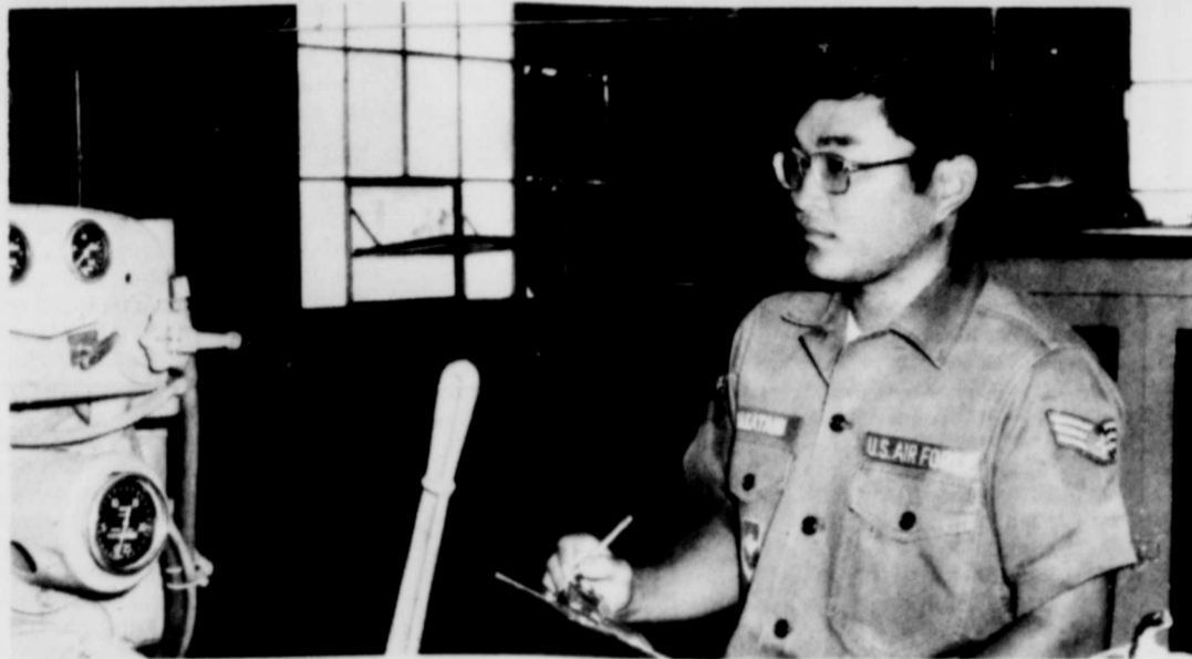
SHEPPARD AFB, TEXAS--WATER PURIFICATION--Sergeant Brian Nakatani examines a diesel pump at the water treatment facility where Sheppard's water is chlorinated, flouridated, and stored. The pump is used in emergencies when there is no electricity for the normal pumps. (USAF PHOTO BY AIRMAN LARRY ORR)
