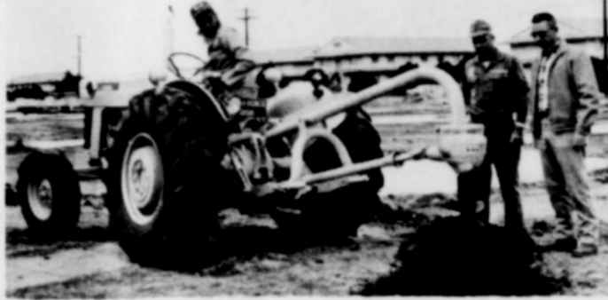
SHEPPARD AFB, TEX.--HOLE IN ONE --Bruce L.B. Shepherd, left, a course supervisor with the Department of Civil Engineering Training of the 3750th Technical School at Sheppard AFB operates a mechanical post hole digger at the site of a new 18 hole miniature golf course here. TSgt. James W. Smith, center, and Ledon G. Bernard, both instructors with the school, watch the action. The miniature golf course scheduled for completion in November, is a self-help project of the department.
