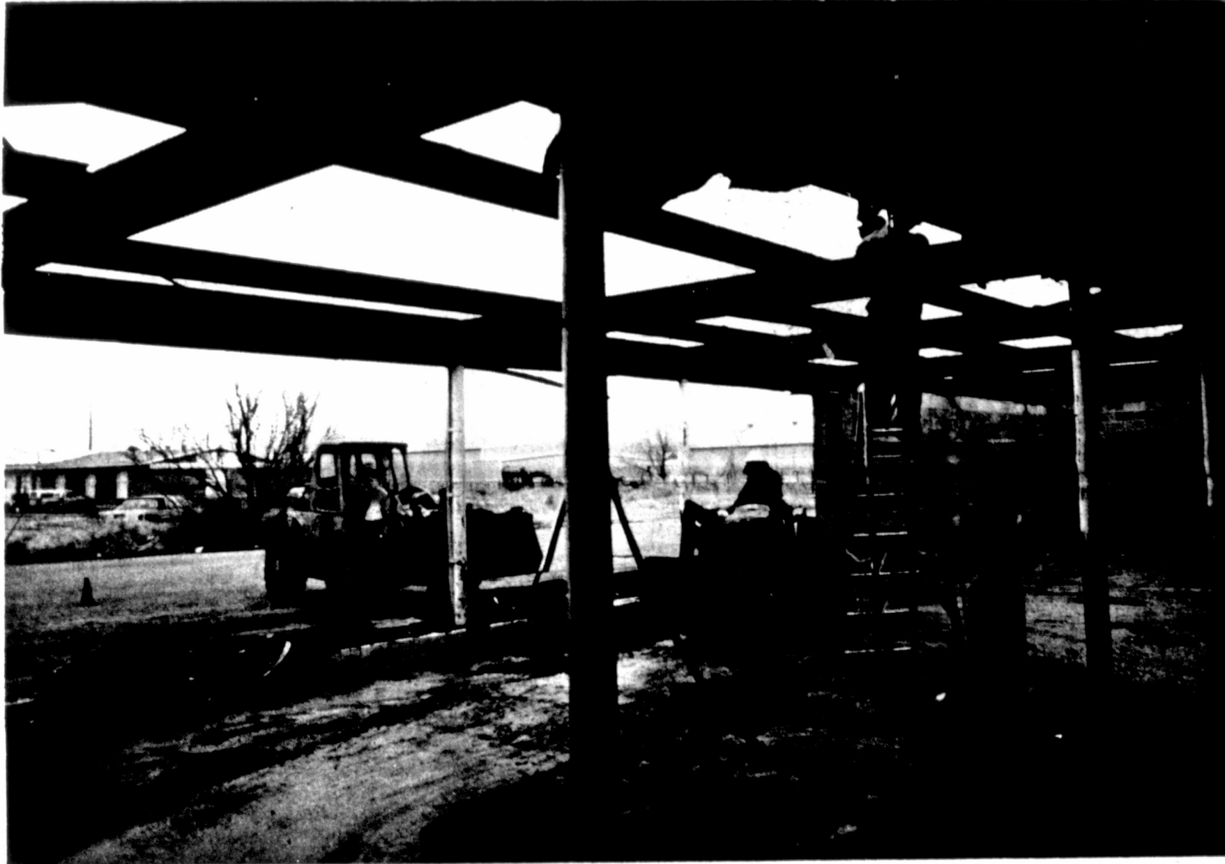
RAISING THE ROOF — Workmen were busy Wednesday afternoon with the early stages of renovating the old Furr's building adjacent to the First Baptist Church in central Snyder. The building will be
