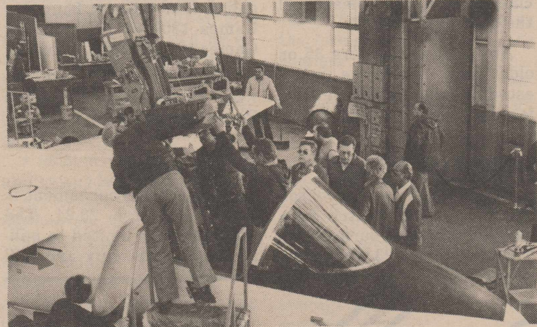
Fairchild Republic Company engineers install an ejection seat in the T-46A pilot trainer aircraft, shortly before the plane is rolled out in Farmingdale, N.Y. The "Next Generation Trainer" is scheduled to replace ATC's T-37 aircraft in 1988.
