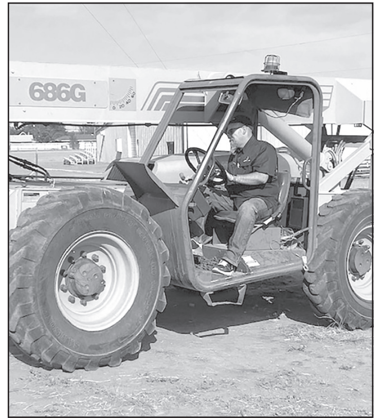
Unloading the pallets
