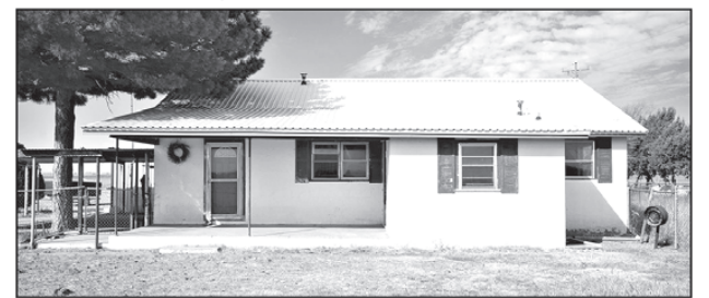
3/1 Stucco Country Home on Highway w/metal roof, approx 8 acres, storage container, carport, fenced yard
