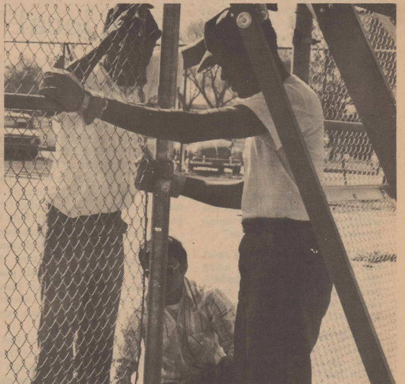
IT'S GOTTA BE TIGHT- (left to right) Theodor Tucker, Ruben Gonzalez and Donald Fuller stretch and anchor the chain link fence around the tennis courts across from the Officer's Club. (U. S. Air Force photo by SSgt. Ron Pack)
