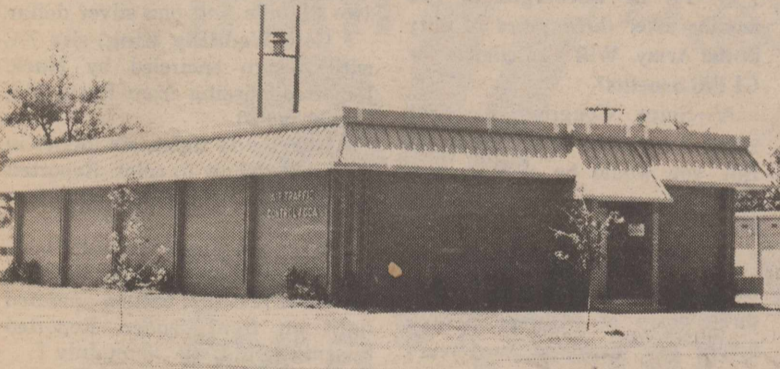
NEW FACILITY — Have you ever passed by this building, behind the 2053rd Communications Squadron building, and wondered what it is? It is soon to be the home of the Comm Squadron's Air Traffic Control
