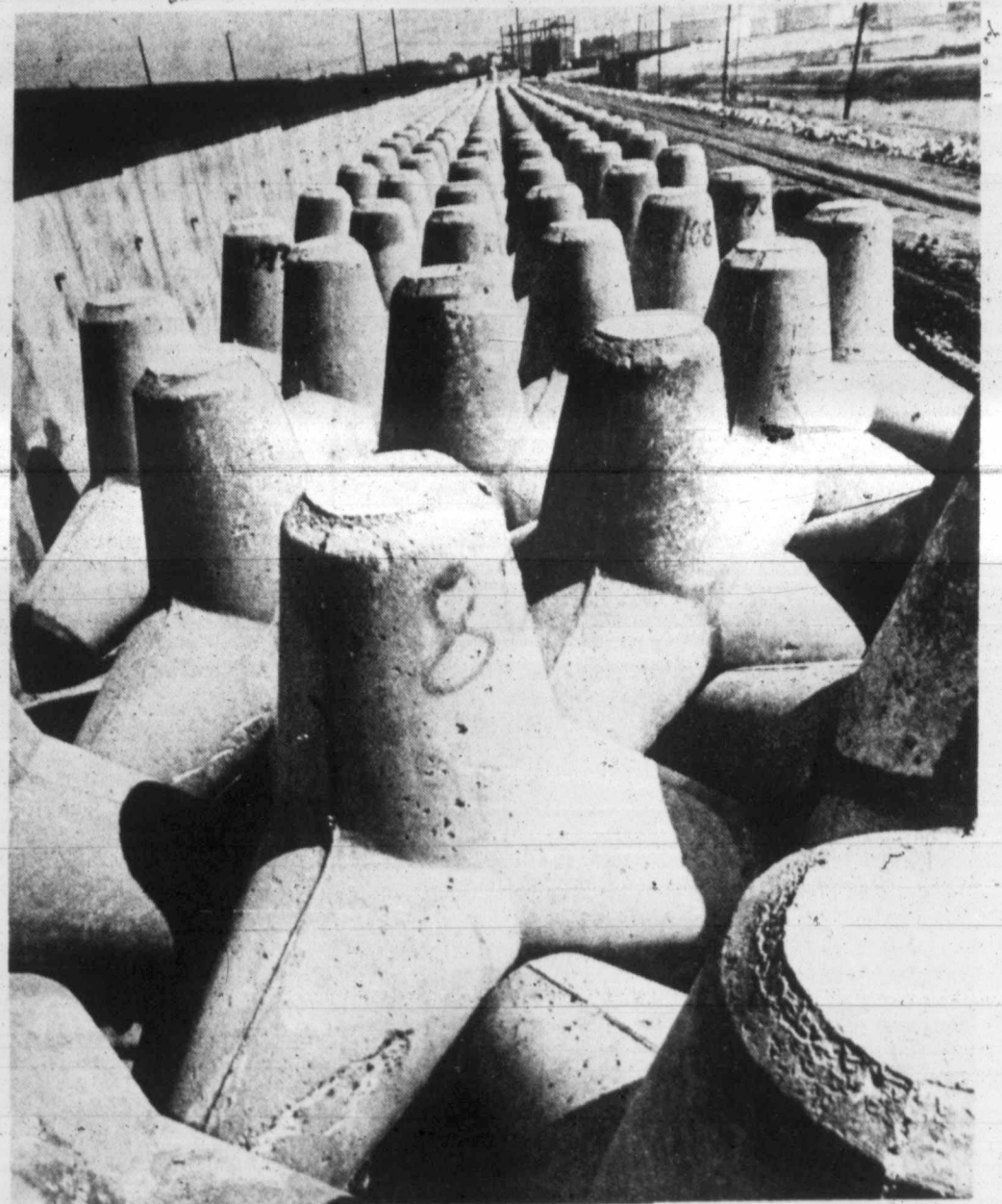
TETRAPODS—Shaped like children's playing jacks, these concrete "tetrapods" are part of a $12 million flood-protection project for the dock area of Exxon USA's Baytown refinery. In the event of a hurricane, the tetrapods would break up the force of heavy waves which might sweep out of a small bay nearby.
