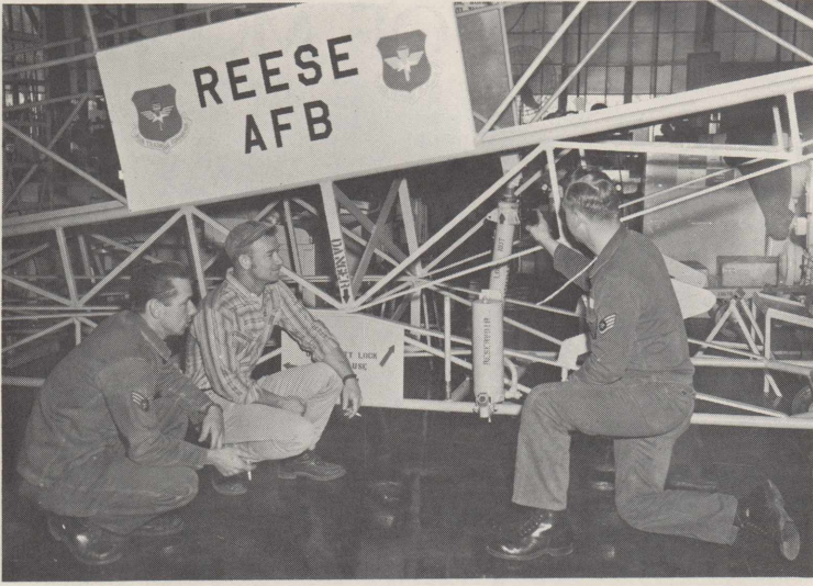
WORK COMPLETED —Reese personnel who designed and built a new medical air evacuation ramp give a final check prior to putting the new equipment into use. SSgt. R. J. Franzen, (right), welding shop supervisor, under whose supervision work was done, takes a look at the hydraulic cylinder as A1C Steve Donald and Civilian Dale Wright, designers and builders, look on.
