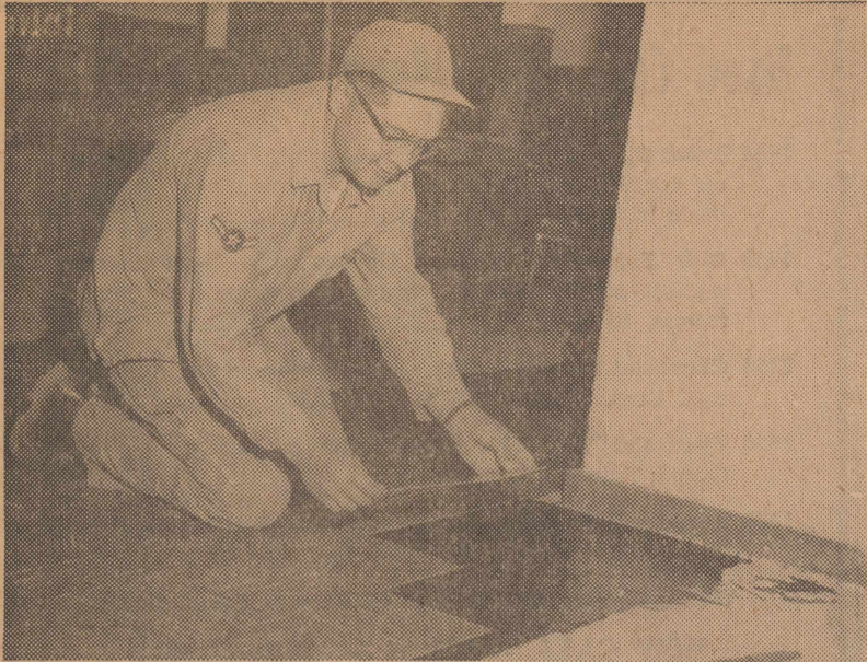
WORK AS USUAL — A/3C Delbert Wilson says he believes work is one of the best things in life to make "a person feel good." Despite completion of a deal to bring him about $58,000 from his tribe's funds, he continues his job as a carpenter at Reese. He's placing floor tile on a floor he just laid. (Photo by Ross.)
