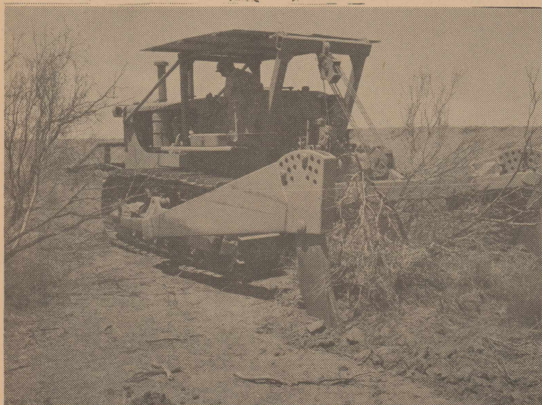
Photo shows the rootplow in operation on the Gordon Cobb ranch located 4 miles southwest of Seminole. The mesquite brush is killed when the blade cuts off the root system at a depth of about 14 inches. The area is then reseeded in the seedbed that has been prepared during the rootplowing operation. A heavy roller-chopper is used to firm the seedbed prior to seeding.
