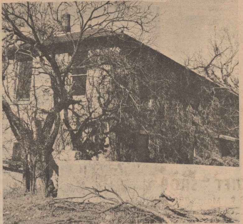
A relay station 20 miles south of San Angelo. The walls are 15 to 18 inches thick, built before 1870.
