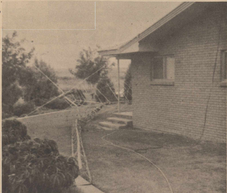
Dr. Alexander's Residence had antenna damage.
