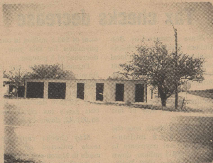
SIX NEW STORAGE spaces will soon be available for lease. Margaret Brunson recently built the spaces on West Main in Bronte.
