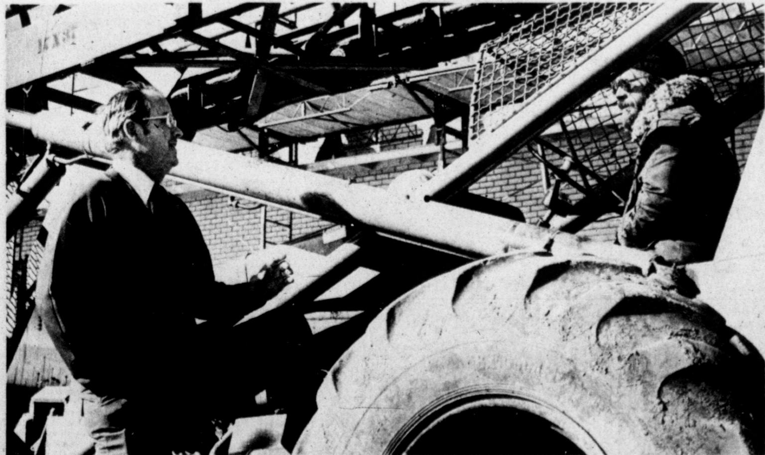
Vitally interested in the future of Midland, Martin Allday, candidate for Mayor of Midland, visits the construction sites of the new mall northwest of Midland.
