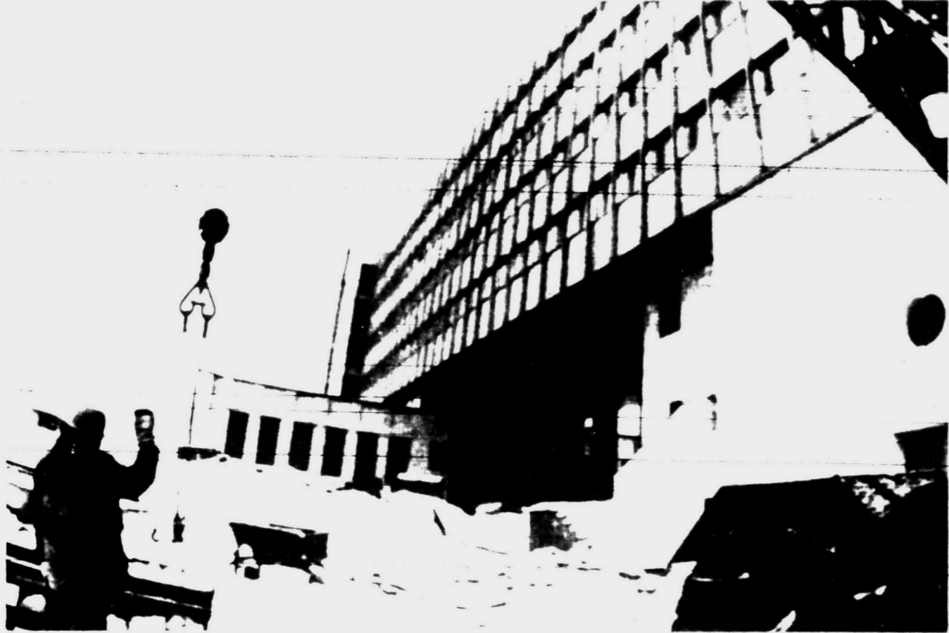
Final construction work proceeds Tuesday on the administration building for Moscow's Olympic Village, the residence center for athletes and officials
